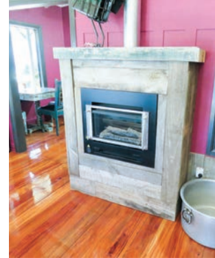
One of two gas fires that back onto each other, with recycled wood surround.
